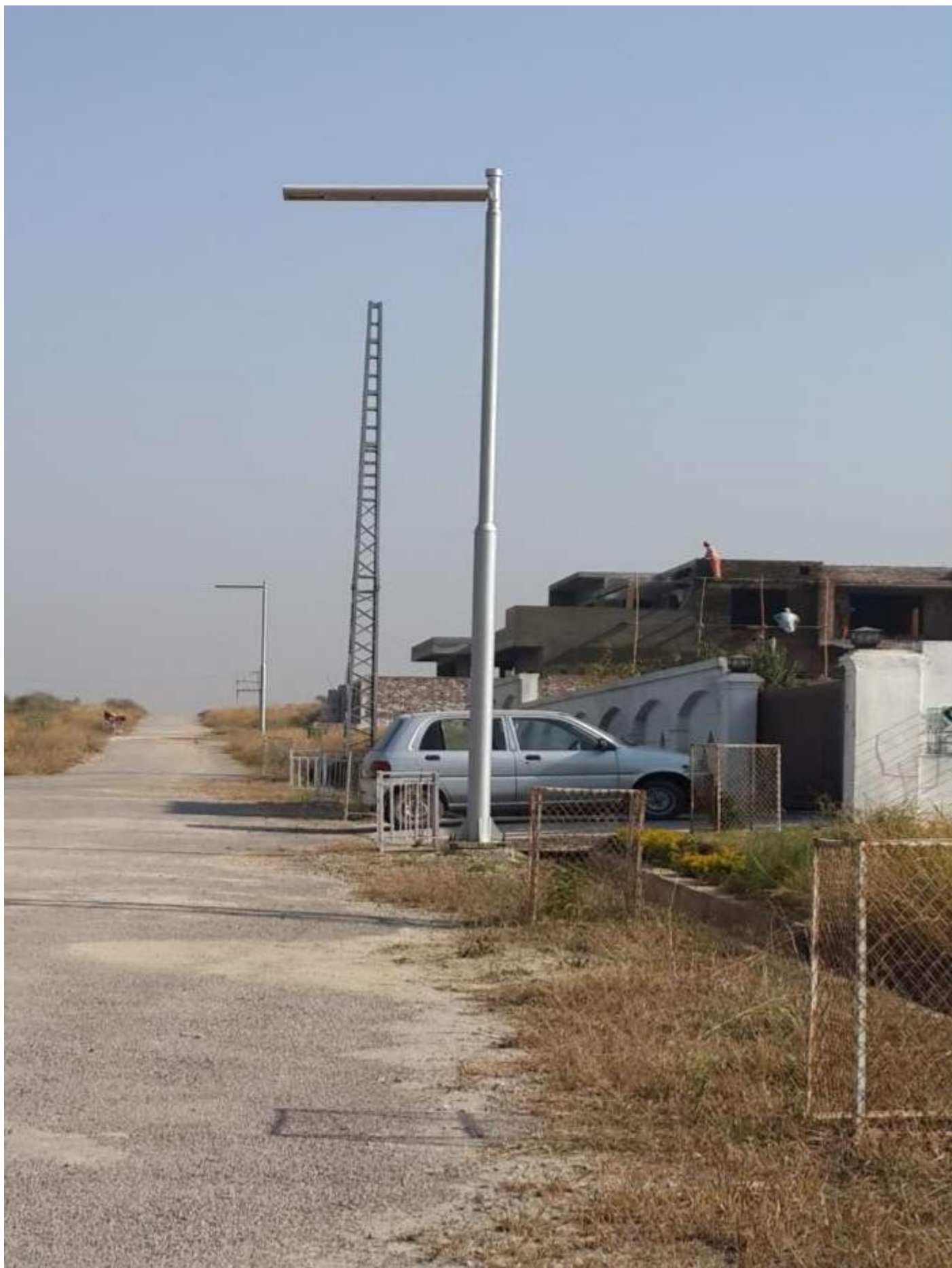
SELF CONTAINED SOLAR STREET LIGHT WITH LITHIUM BATTERY & GLASS LESS PANELS AT ECHS, D-18 ISLAMABAD
