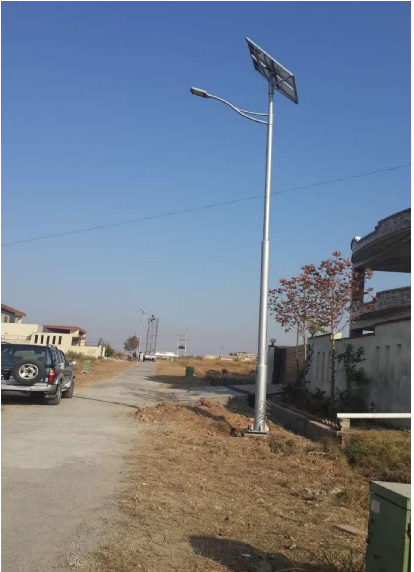
SOLAR STREET LIGHT WITH LITHIUM BATTERY AT ECHS, D-18 ISLAMABAD
