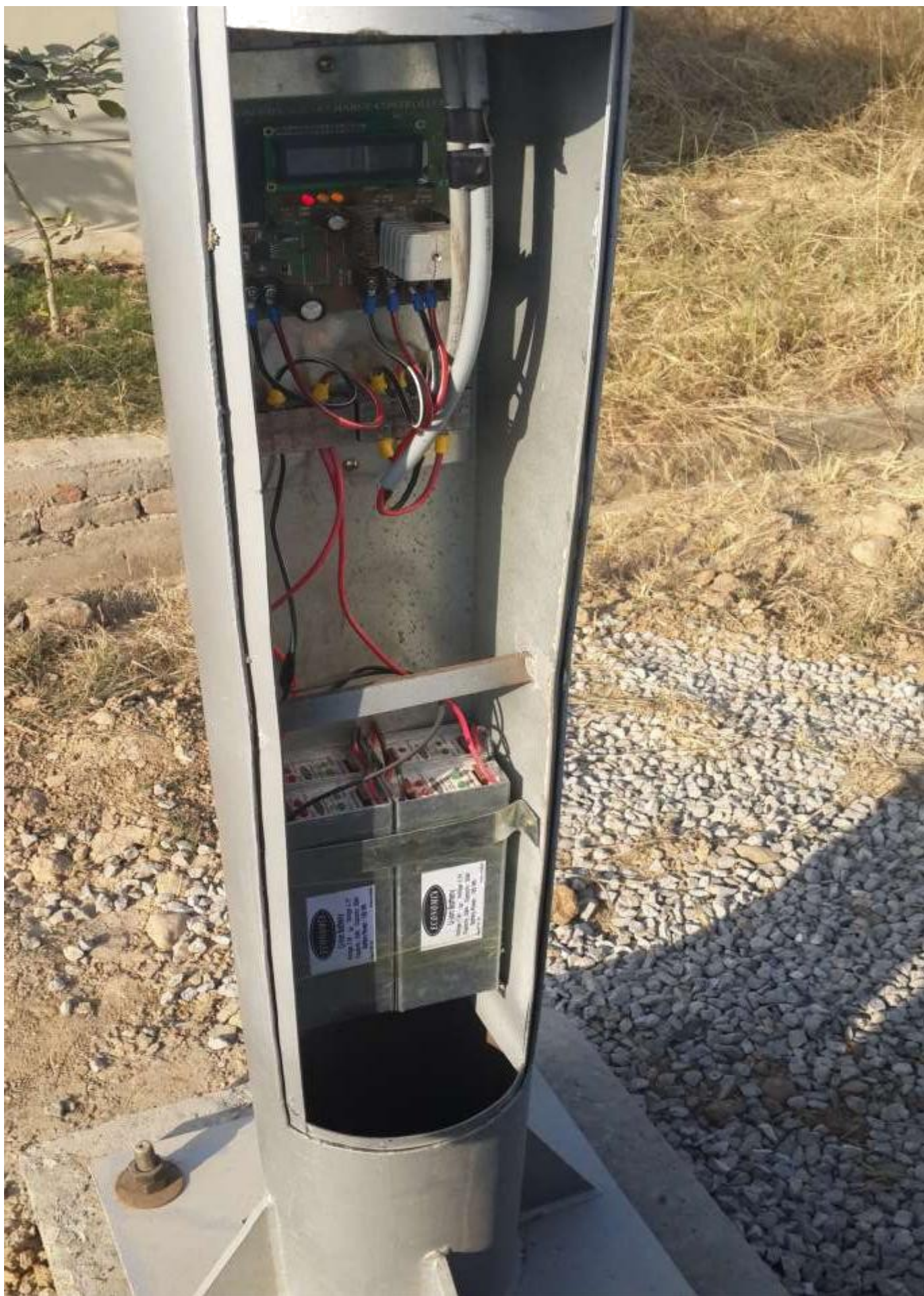
SOLAR STREET LIGHT WITH LITHIUM BATTERY AT ECHS, D-18 ISLAMABAD
